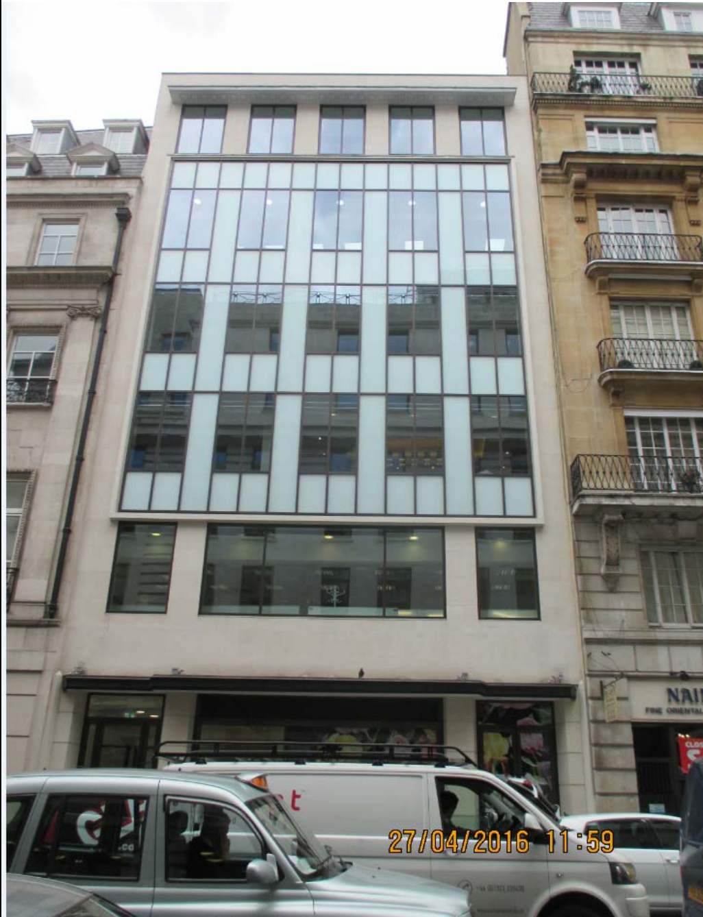
Front elevation of application site
